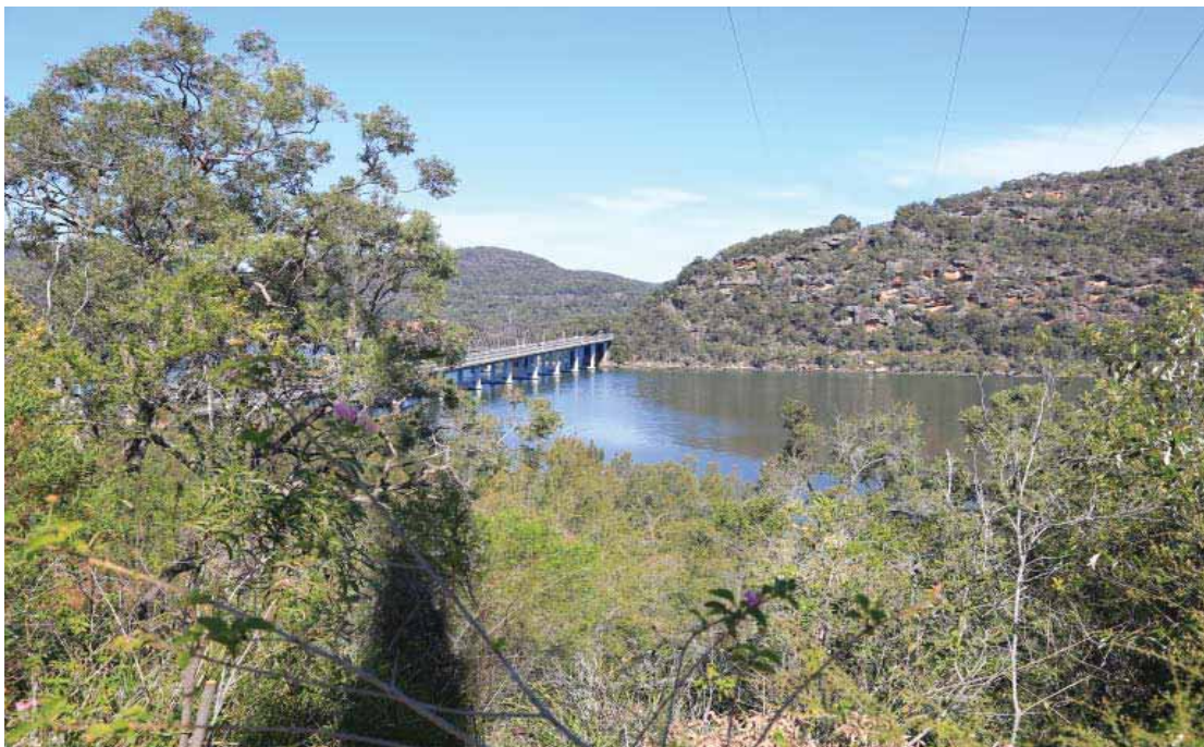
Plate 12 View south from vantage point on brow of hill proposed for future public recreation use at south end of site
